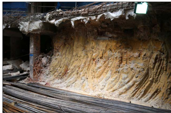
Figure 6: Face of excavated soil exposed during Basement Excavation
