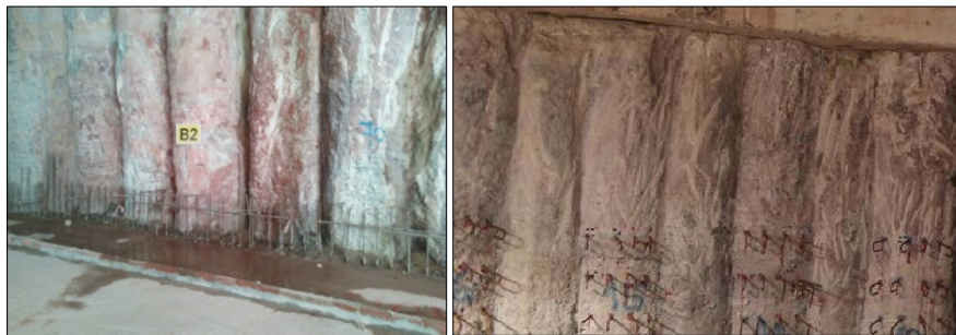
Figure 12: Exposed View of CBP Wall (left) and SBP Wall (right)
