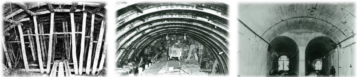
Figure 7: Photos showing timber lagging, curved rails and concrete lining used in double track tunnels in the City of Sydney railway tunnels (Fraser, 1930).
