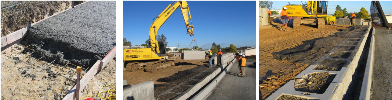
Figure 5: Installation processes of Stone Strong blocks wall and geogrid reinforcement
