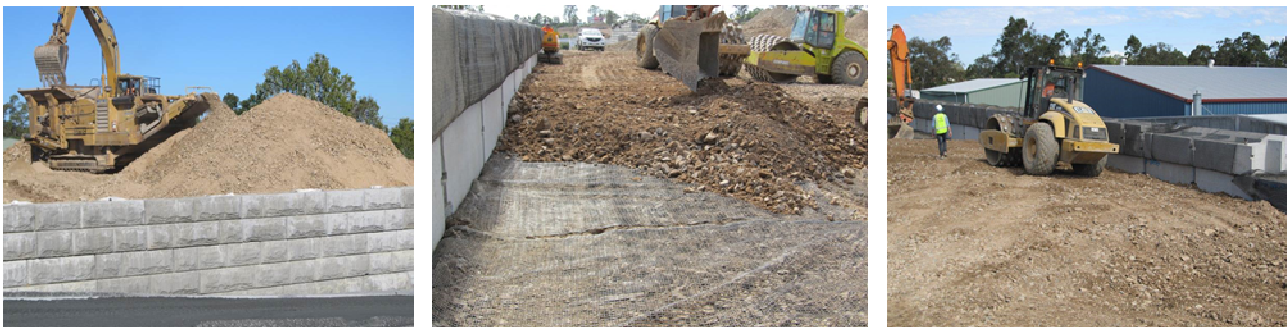
Figure 8: Construction processes of adopting in-situ materials
