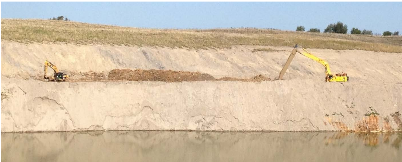
Picture 7: Barrier Wall being excavated through dragline spoil
