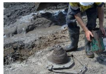
Picture 1: Slump Testing
