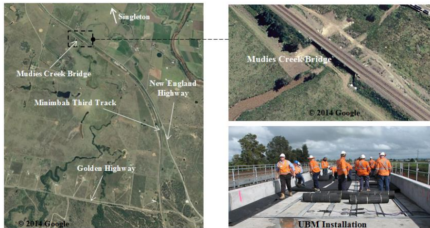
Figure 31: Mudies Creek Bridge Location and Installation of UBM (sourced from Indraratna et al. (2014))
