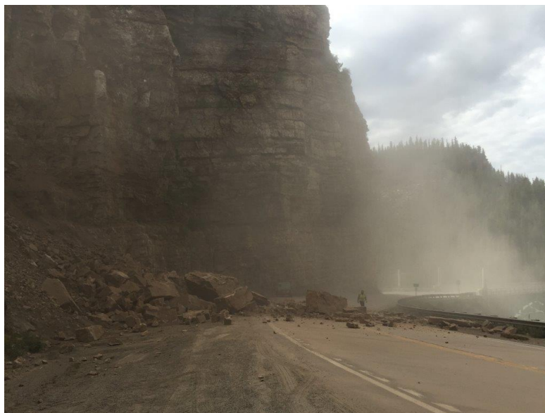
Figure 5: Rock Slope Risk Exposure Reduction on US 24 near Minturn, Colorado.
