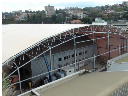
Figure 14: The OCE under construction (over the top of Building No. 11).
