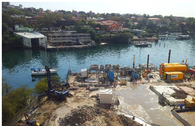
Figure 12: Jet Grouting on the seawall after initial trials.
