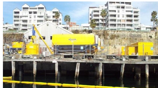
Figure 11: Jet Grouting support plant on the wharf.
