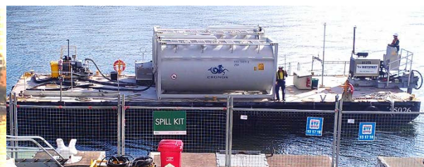
Figure 10: Cement supplies arrived daily by barge.
