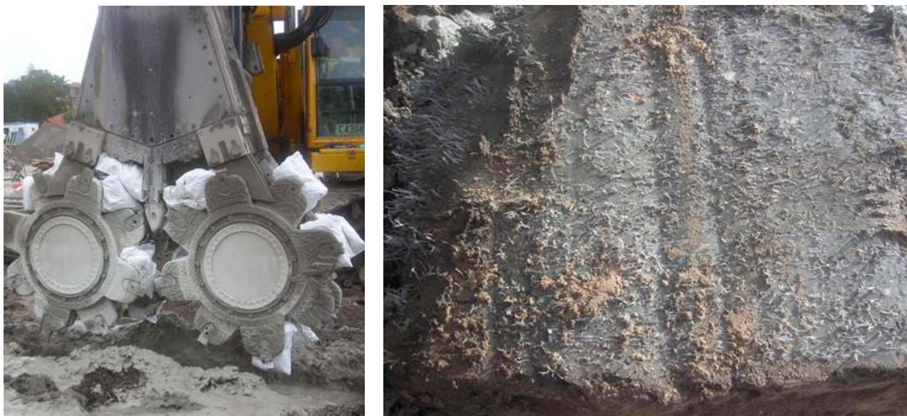
Figure 1: Fibres in paper bags add to the cutter (left). Surface of soil fibre mix showing effective mixing and dispersion (right)
