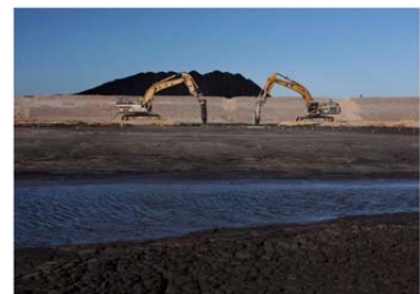
Mass Soil Mixing at NCIG - Keller Ground Engineering
