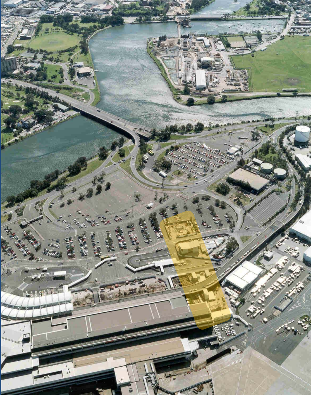
View to and from the International Terminal, Sydney Airport
