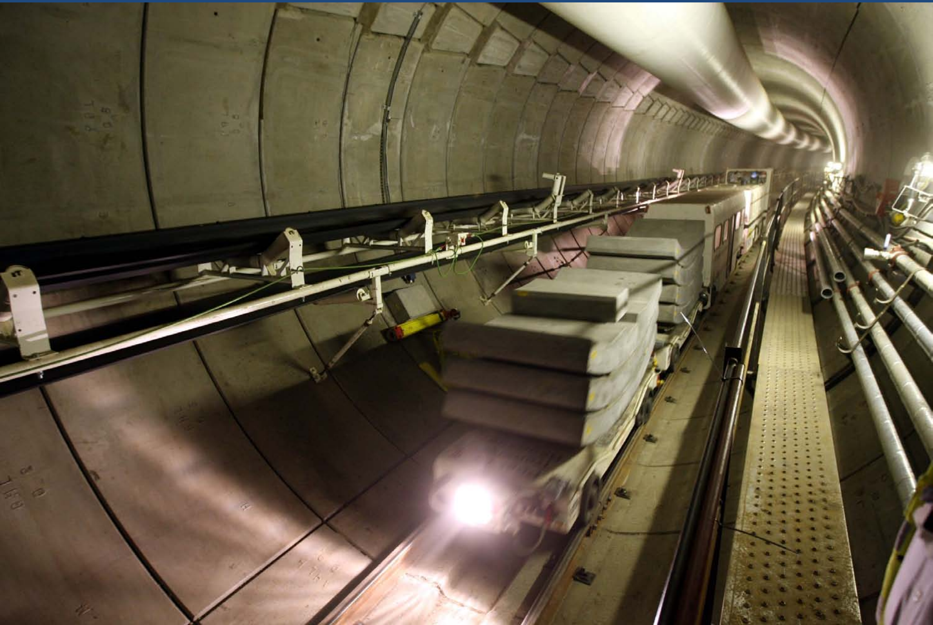
Baggage Transfer Tunnel
