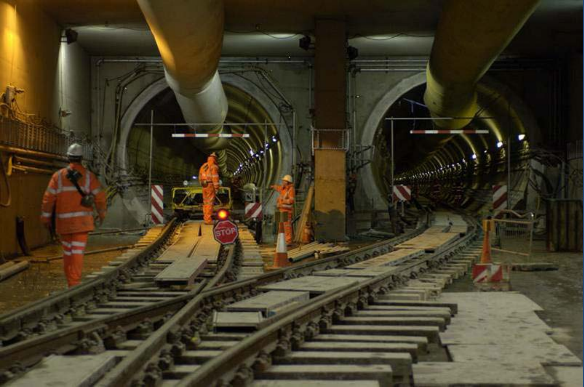
Piccadilly Railway Tunnels
