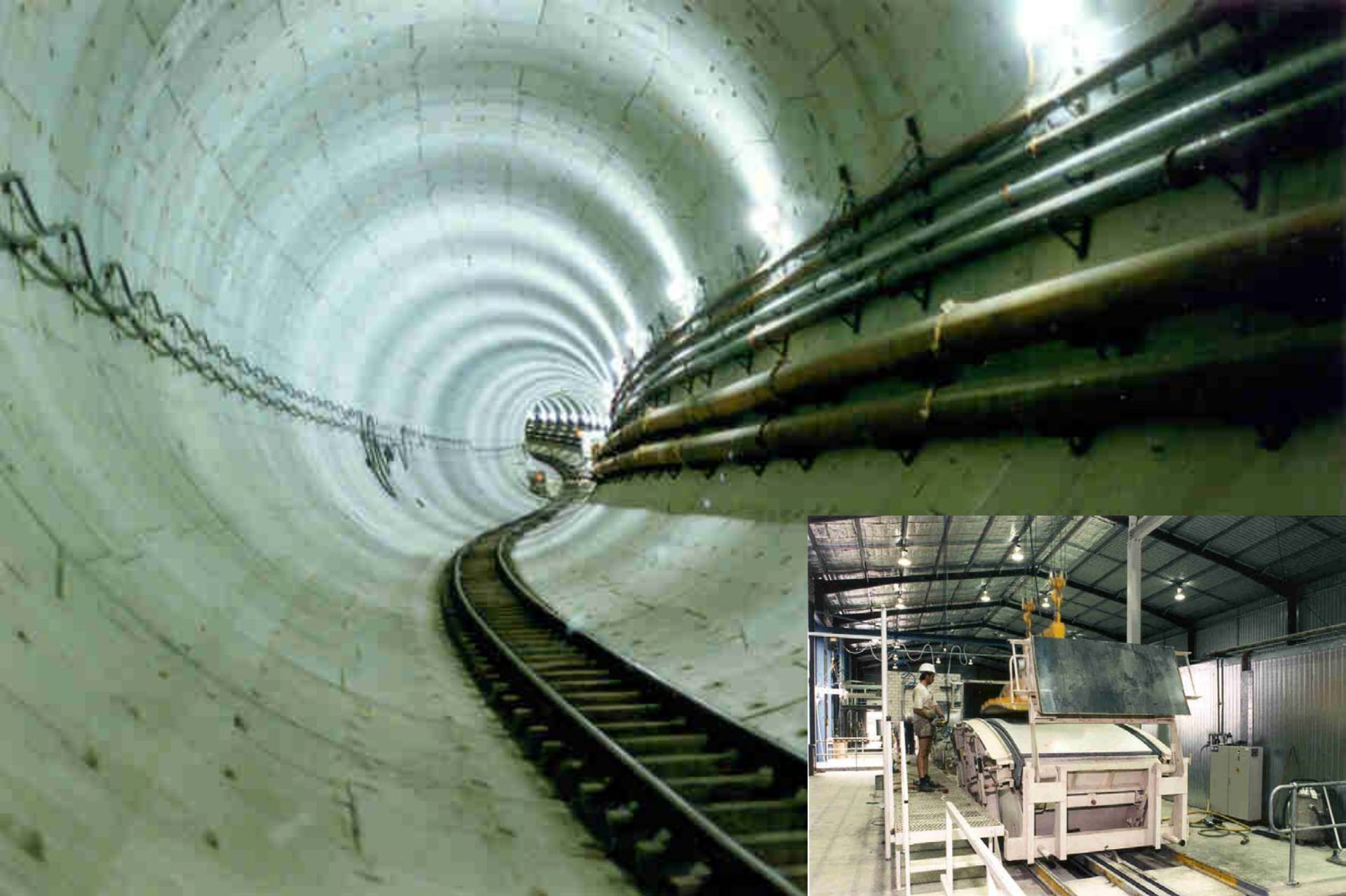
Soft Ground Tunnel - Watertight Concrete Segmental Lining
