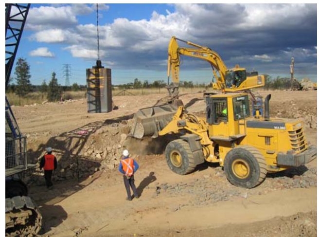
Photo 8: Backfilling of DC hole.
