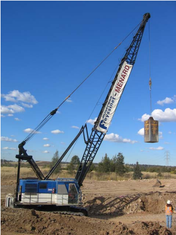
Photo 5: Dynamic replacement (DR).
