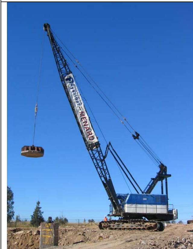
Photo 3: Dynamic compaction (DC).
