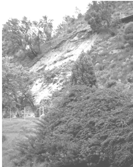
Figure 4: Shallow slope failure in yellow sand over Tamala Limestone at Kings Park.
